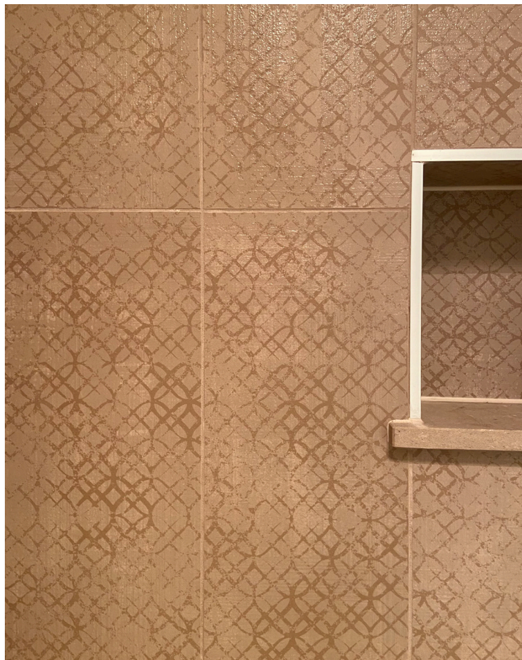
Project 3044. Etro Matt Hazelnut laid in vertical stack on shower wall.
